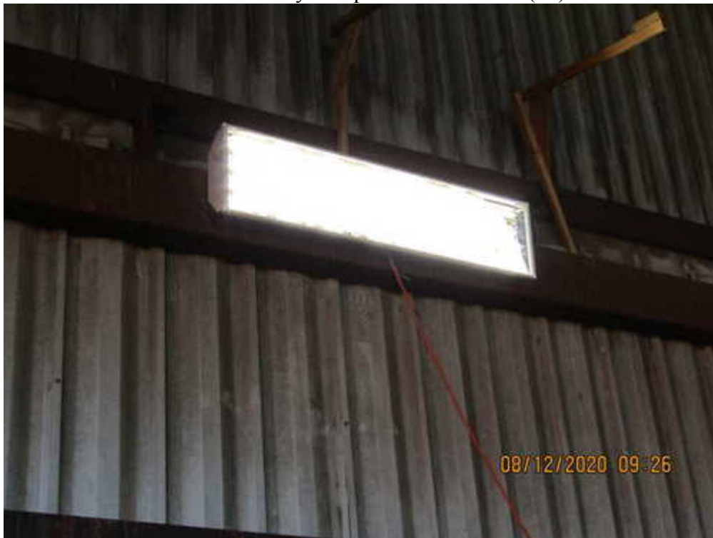
5770 N Industrial Pkwy - Inspection 8-12-2020 (26).JPG
